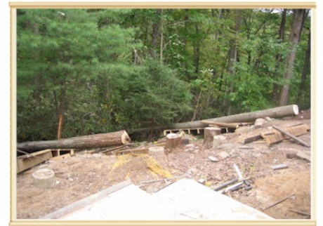
The Ongoing Construction Project
