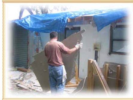
Tearing Down the Old Kitchen
