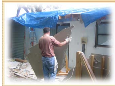
Tearing Down the Old Kitchen
