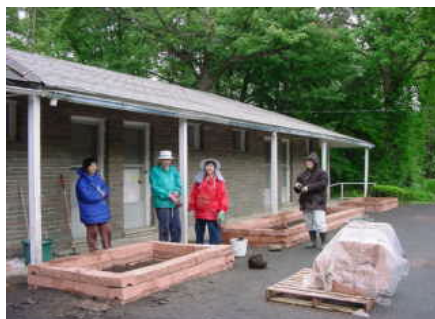
The completion of building the outer walls for the flowerbeds
