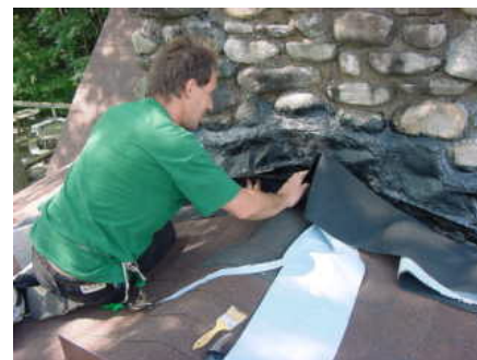
Fixing the chimney
