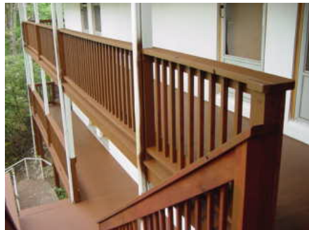
Painted staircase at the back of the Retreat House
