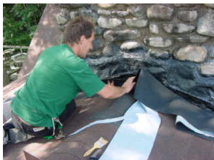
換修屋頂補煙窗
